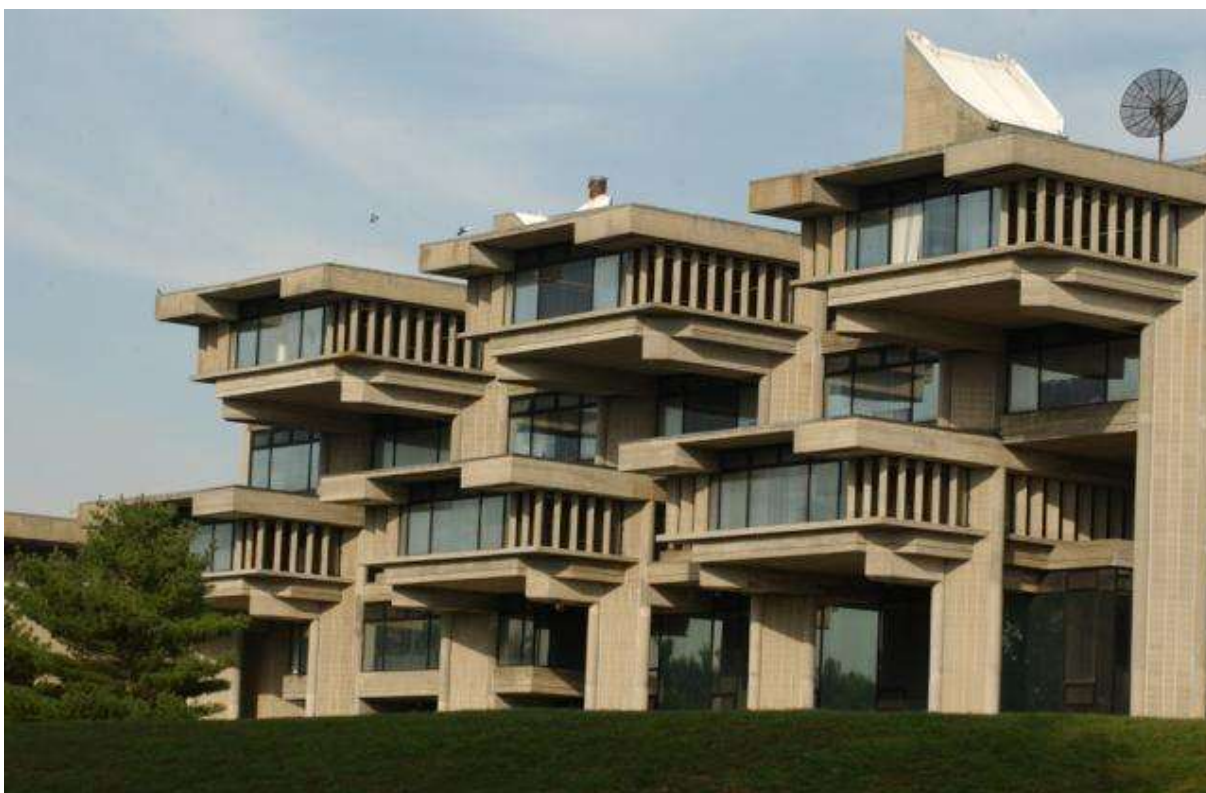
Obr. 5 Detail fasády, zdroj: Claire T. Carney Library, Paul Rudolph & His Architecture: http://prudolph.lib.umassd.edu/home Odečteno 15. 11. 2014
