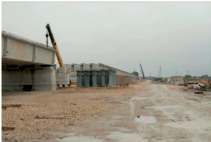
Figure 3: Construction Site, photograph by the author
