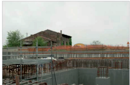
Figure 4: Construction Site, photograph by the author
