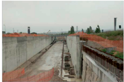
Figure 2: Construction Site, photograph by the author
