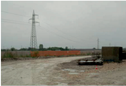
Figure 1: Construction Site, photograph by the author
