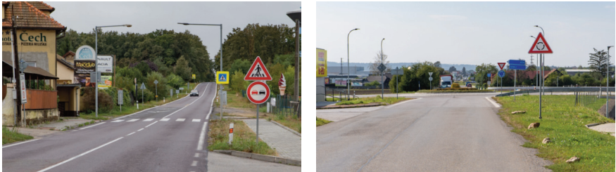
Figure 8: Warning signs placed in close proximity to the "danger"
