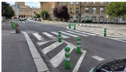
Figure 17: Reducing intersection size with road markings and bollards.
