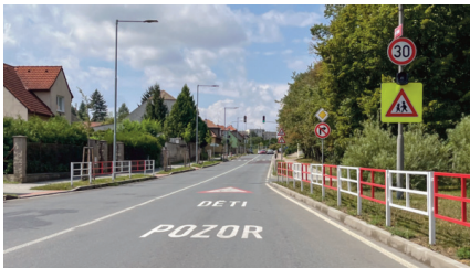
Figure 21: Visual pollution from excessive signage and railings near a traffic light.
