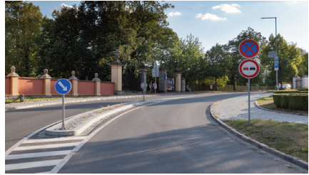
Figure 10: Anomalous and irrelevant use of overtaking signs in built-up area
