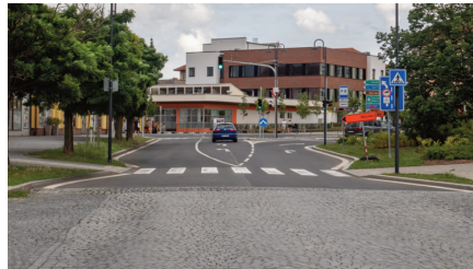
Figure 20: Missed opportunities to build a pedestrian crossing island.
