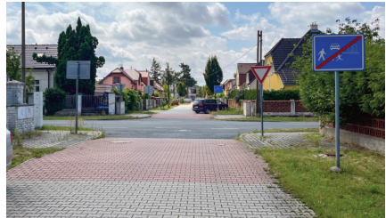
Figure 12: Unnecessary give way signs at the end of a home zone.
