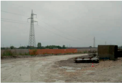
Figure 1: Construction Site, photograph by the author
