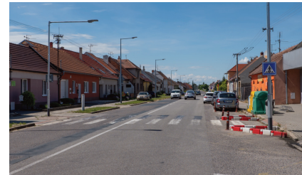
Figure 19: Permanent shortening of pedestrian crossing using temporary measures.
