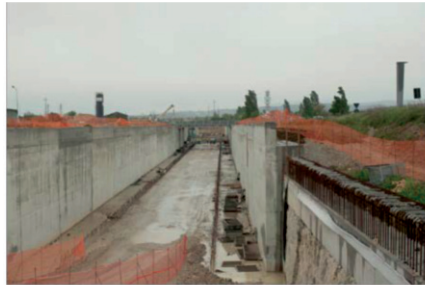
Figure 2: Construction Site, photograph by the author
