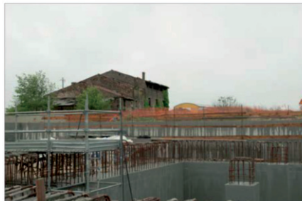
Figure 4: Construction Site, photograph by the author
