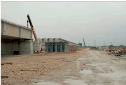
Figure 3: Construction Site, photograph by the author
