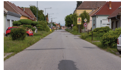
Figure 24: 7.0 m wide road without road markings
