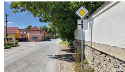
Figure 11: Redundant additional plates showing standard intersection diagram.
