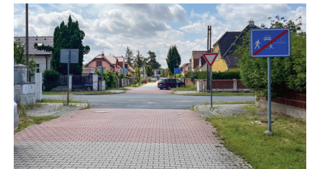
Figure 12: Unnecessary give way signs at the end of a home zone.
