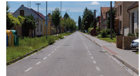
Figure 25: 7.7 m wide road with protective cycle lanes
