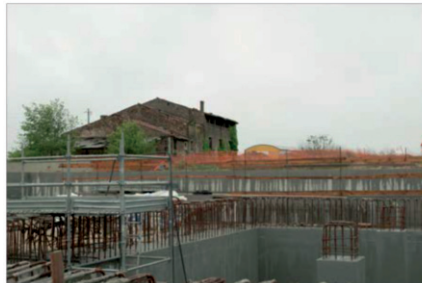
Figure 4: Construction Site, photograph by the author
