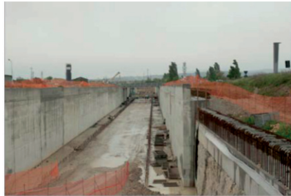
Figure 2: Construction Site, photograph by the author
