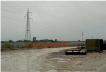
Figure 1: Construction Site, photograph by the author
