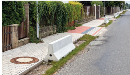
Figure 16: Prohibited parking in purposeless stripe of a street.
