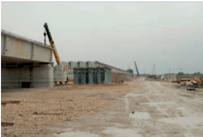
Figure 3: Construction Site, photograph by the author
