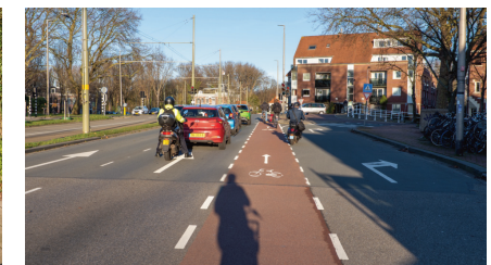
Figure 6: 4-lane arrangement in the Netherlands with no erected traffic sign.
