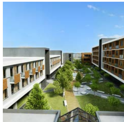
3A Monash University, vnitroblok
