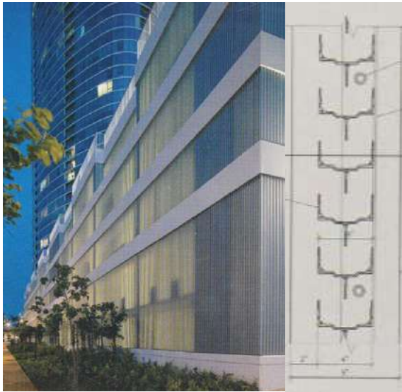
Obr. 34 - Moana Pacific Condominium Tower, Honolulu (2005)
