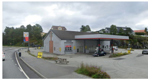
Figure 55.) Gas station Source: streetview google earth
