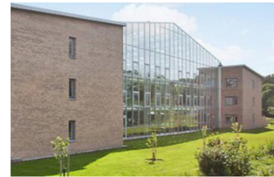
Figure 9.) Structure in daylight [21]
