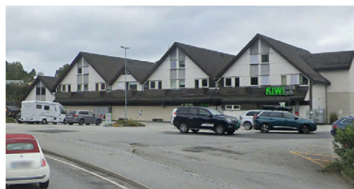
Figure 56.) Sagvågsgården Source: streetview google earth
